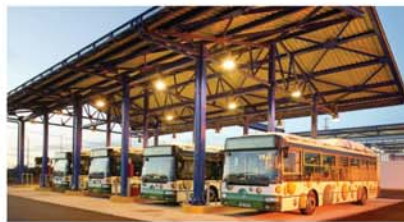
CNG Refueling Station in Anthousa, Attica
