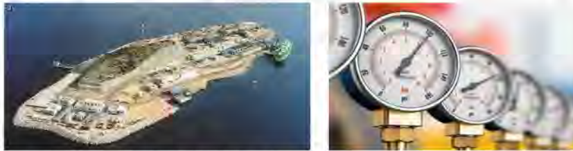
Terminal for Liquefied Natural Gas (island of Revythoussa)
