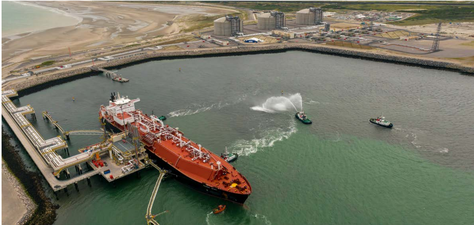
Dunkirk LNG Terminal First Delivery – Courtesy TOTAL
